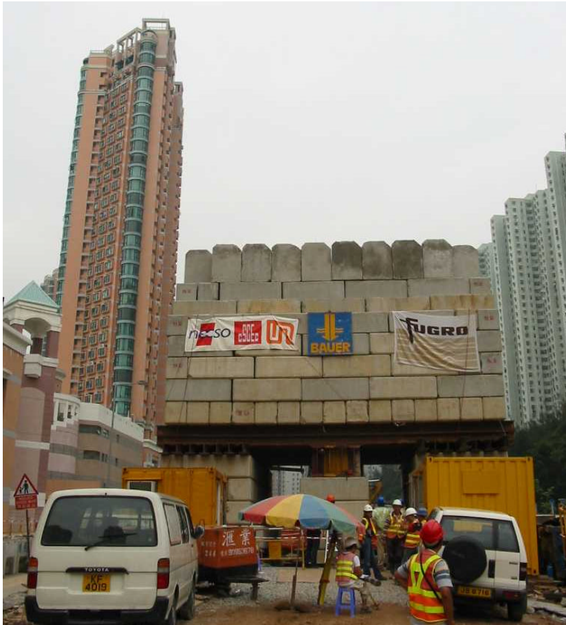
Pile load test in progress in Ma On Shan town centre
