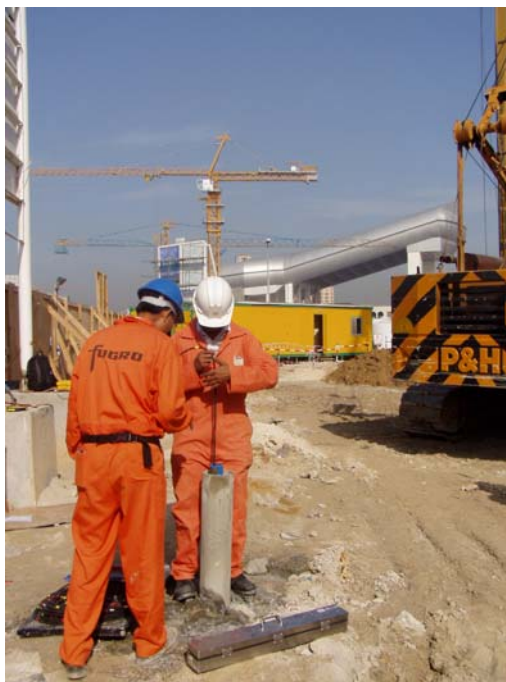
Inclinometer Reading Prior to Excavation
