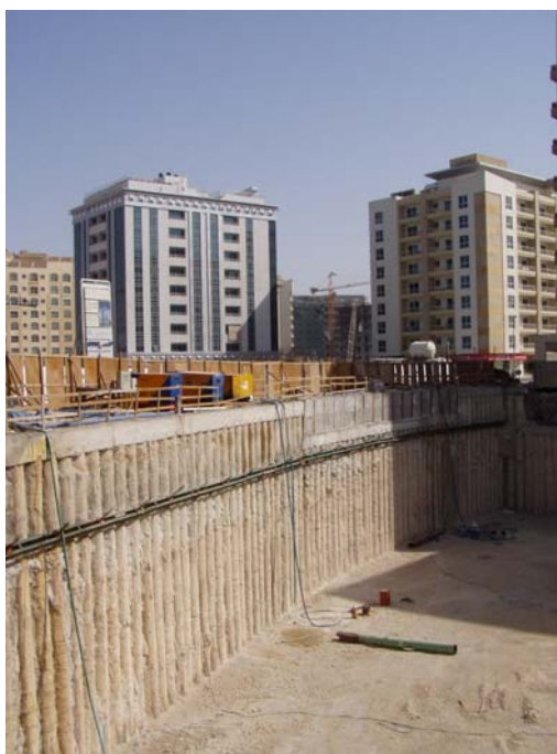
Final Excavation Level
